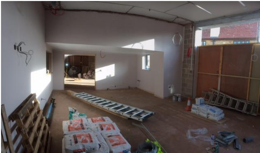
Picture 5. Large office looking towards the entrance hallway
