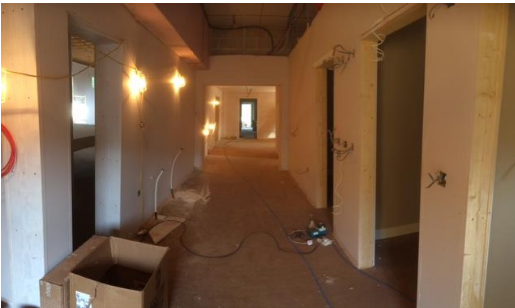
Picture 6. Entrance from Car Park
