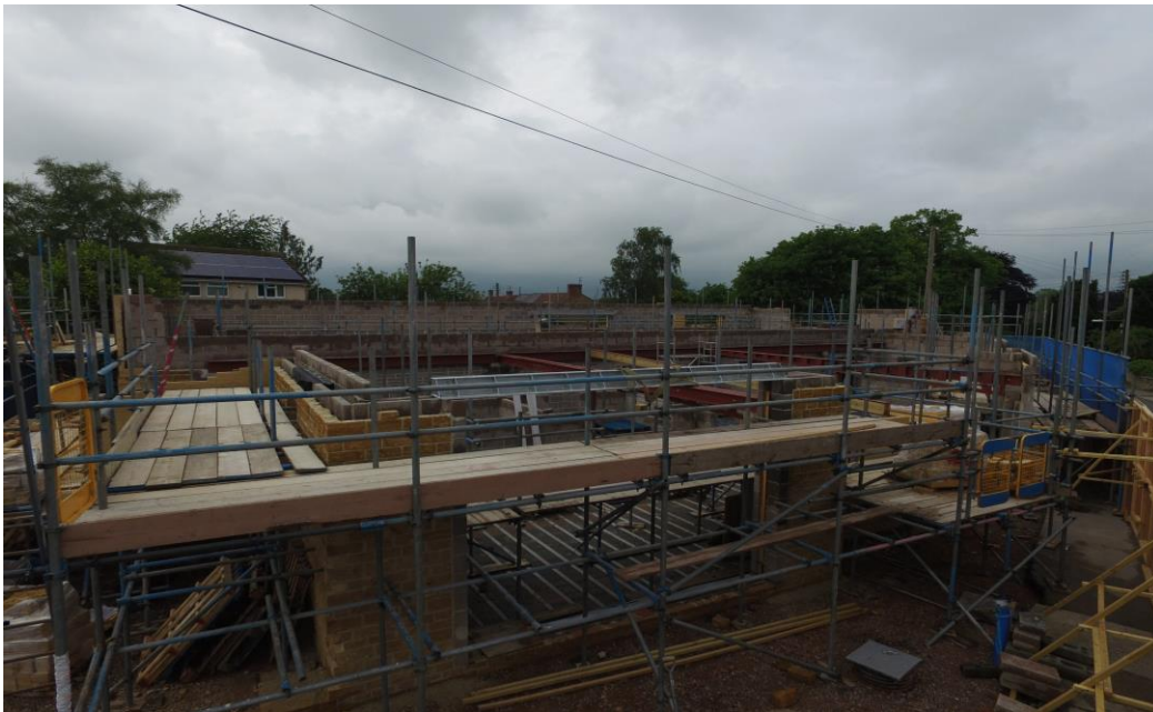
Photo. 3 ` Showing special reinforced galvanised lintel over wide window aperture
