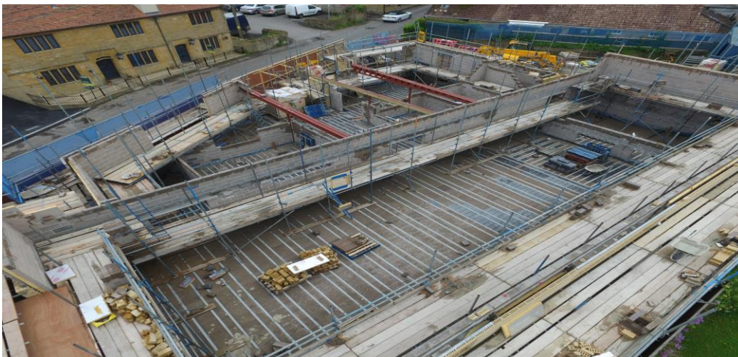
Photo 2. Above the main hall looking towards the public highway
