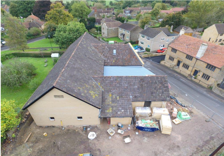
Picture 1 . Showing roof coverings , including Zinc and Scaffold removed
