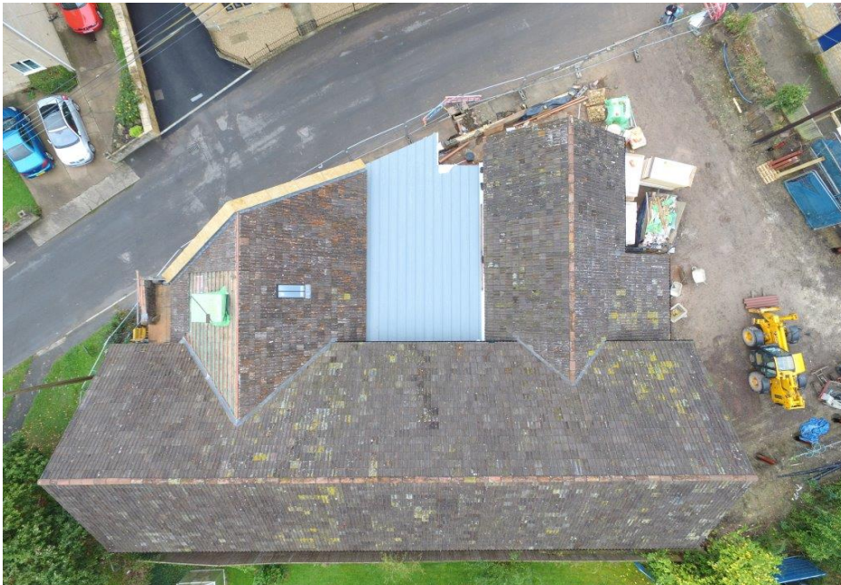
Picture 3. Aerial view showing roof coverings and hamstone chimney installed (wrapped in polythene)
