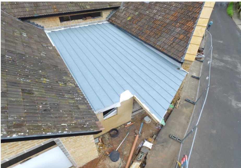
Picture 2. Showing the standing seam zinc roofing
